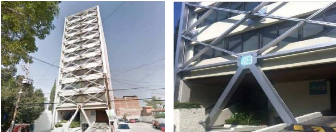
Figure 1.7: Retrofit intervention with 2D// steel exoskeleton of the Hospital Ángeles Clínica Londres in Mexico City [11].
