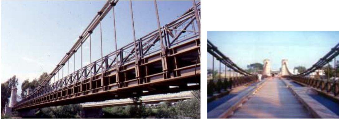
Figure 2.11: The Real Ferdinando Bridge on the Garigliano River, Italy [8].
