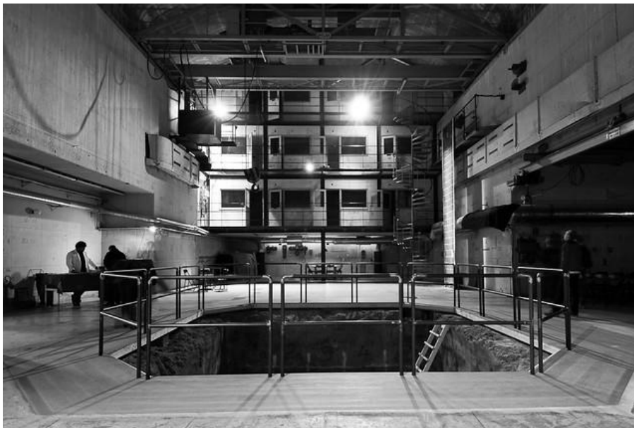
Figure 19: Former nuclear reactor R1, now a research center and art space of KTH campus in Stockholm, Sweden (source: Green Hackathon.com)
