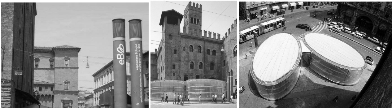
Figure 9 - the former Urban Center, Ebo located in Re Enzo square. Source: La Repubblica 2003
