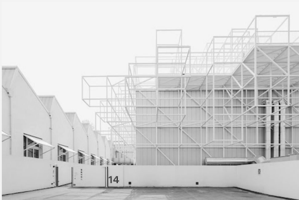
Figure 50 - The New Center for The Arts at Opificio. Photo: G. De Vincentis
