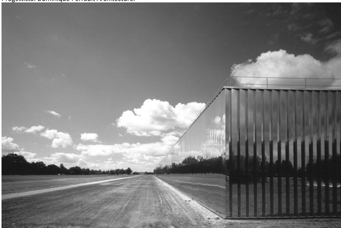
Aplix factory (1999), Le Cellier-sur-Loire, Francia. Progettista: Dominique Perrault Architecture.
