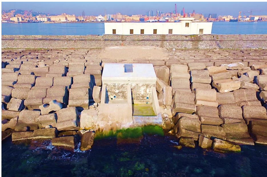
Figure 53. The OBREC prototype installed in the San Vincenzo breakwater, port of Naples.
