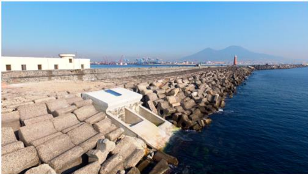
Figure 24. OBREC prototype installed in the port of Naples.
