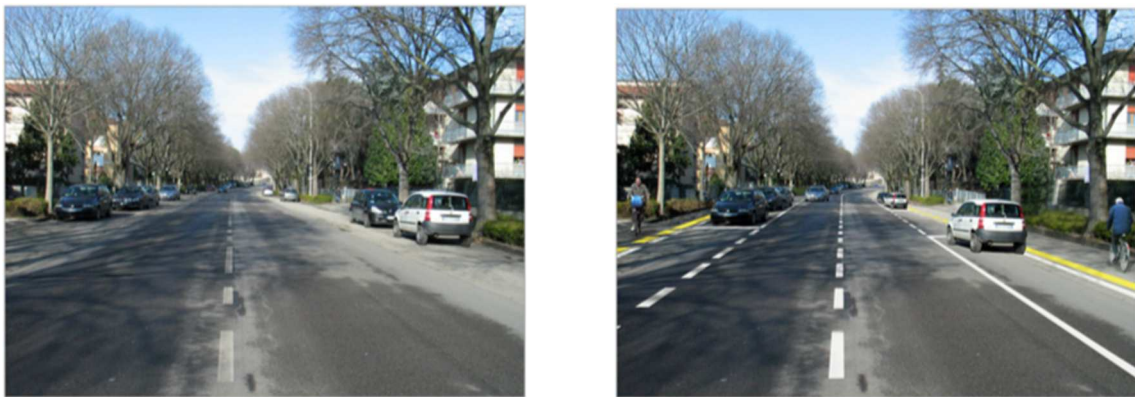
Figure 22. Narrowing the street before and after the intervention
