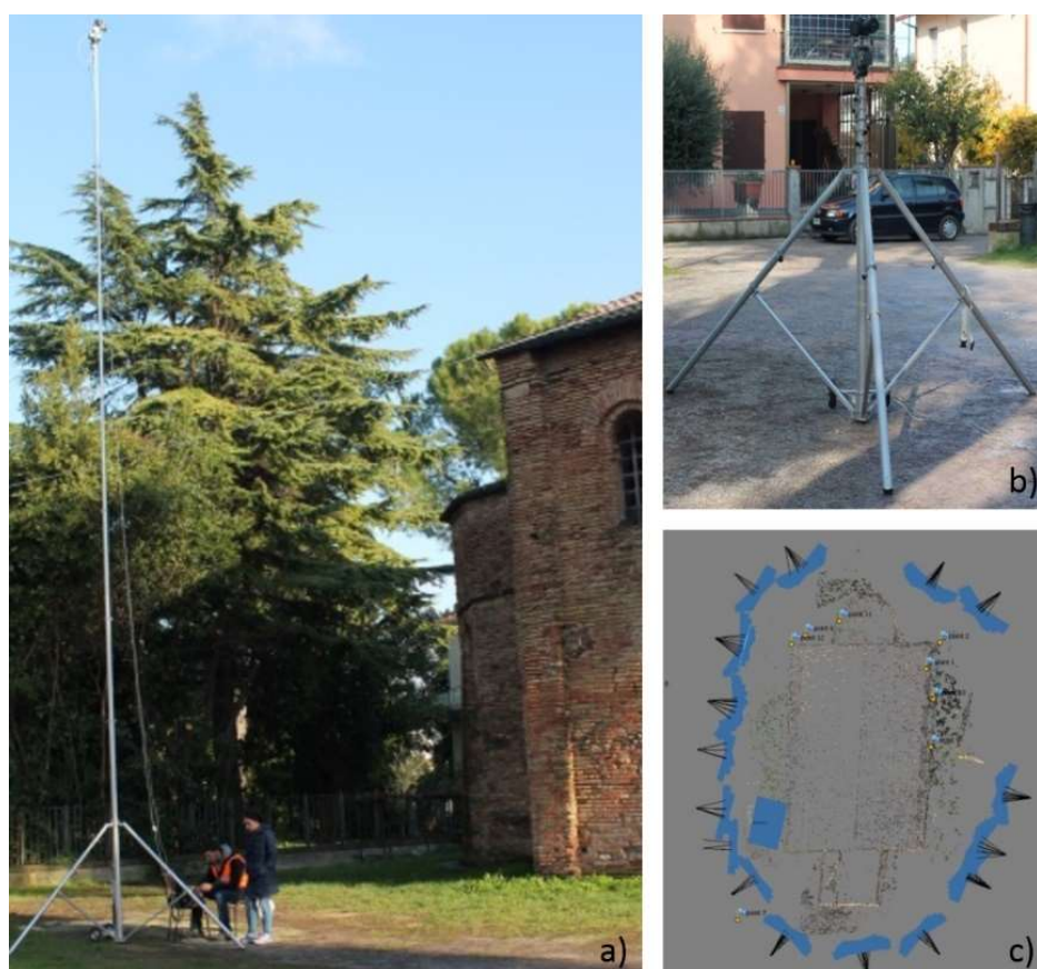
Figure 45. The photogrammetric survey of the church roof: a) and b) equipment used for the images acquisition, c) reconstruction of exterior orientation after the image alignment phase in the SfM processing
