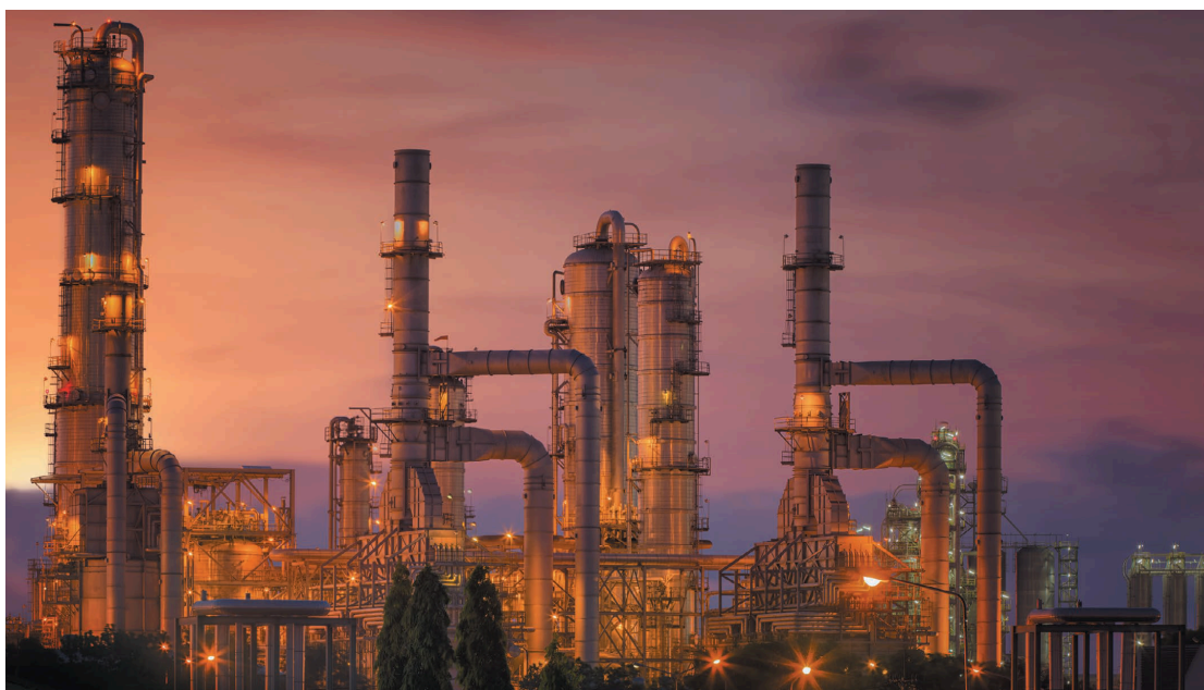
Figure 2.3: Chemical plant from source [19] .
