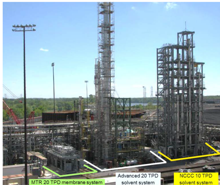
Figure 3.7: Representation of the compactness of membrane technologies compared to other competitive technologies for carbon capture. 20 tons per day membrane system by MTR (green), amine absorption columns 20 tons per day (green), and 10 tons per (yellow). [60]
