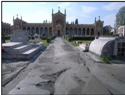
Figure 1 Liquefaction sand boils developed during the 2012 Emilia earthquake in the cemetery located in Sant'Agostino (Lo Presti et al., 2013).
