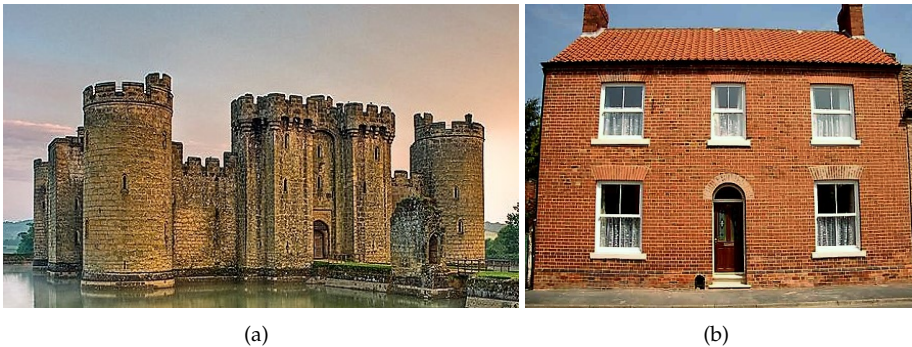
Figure 1: Examples of (a) monumental and (b) ordinary masonry structures.
