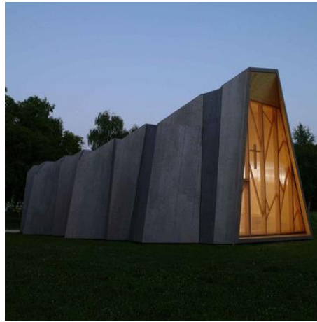
Figure 99: temporary chapel for the Deaconesses of St-Loup, Localarchitecture + Danilo Mondada.
