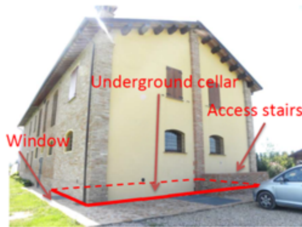
Figure 4.54: Picture of the farm building with the indication of the underground wine cellar location.
