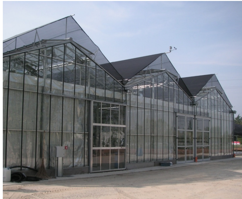
Figure 2.3: Picture of a double-pitched greenhouse with several spans, of an experimental structure of Unibo, in Imola.
