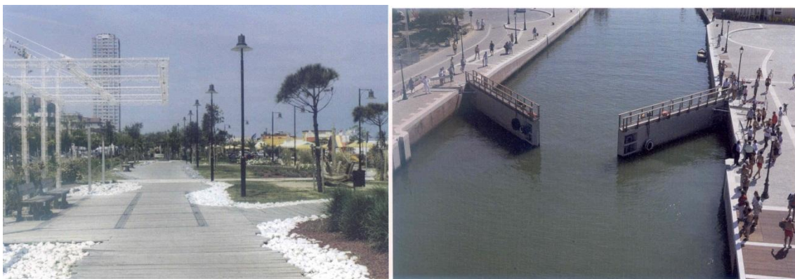
Figure 10 Mitigation measures: the “Gardens of Cesenatico”: dike behind bathing facilities; sea gate in correspondence of the Canal Harbour.
