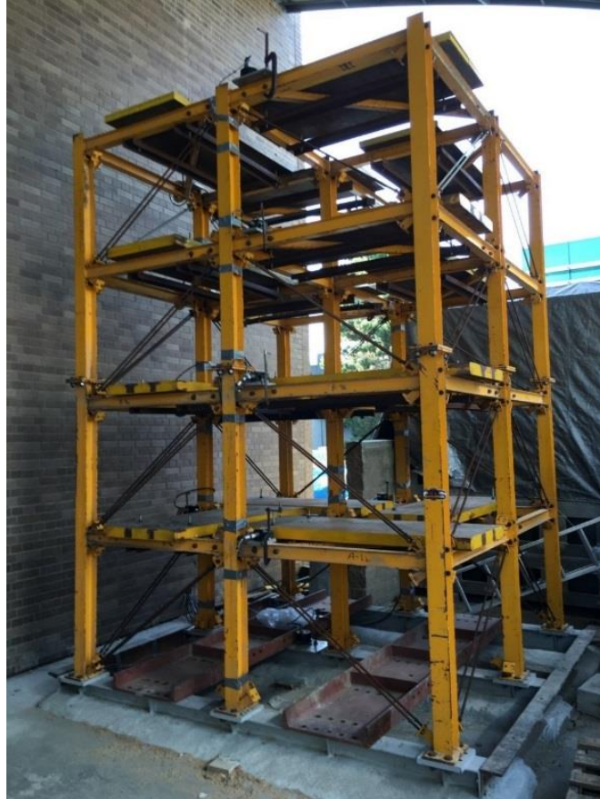
Figure 5.3. Steel frame structure (EERF laboratory, UBC) [Bernagozzi et al., 2017 b]
