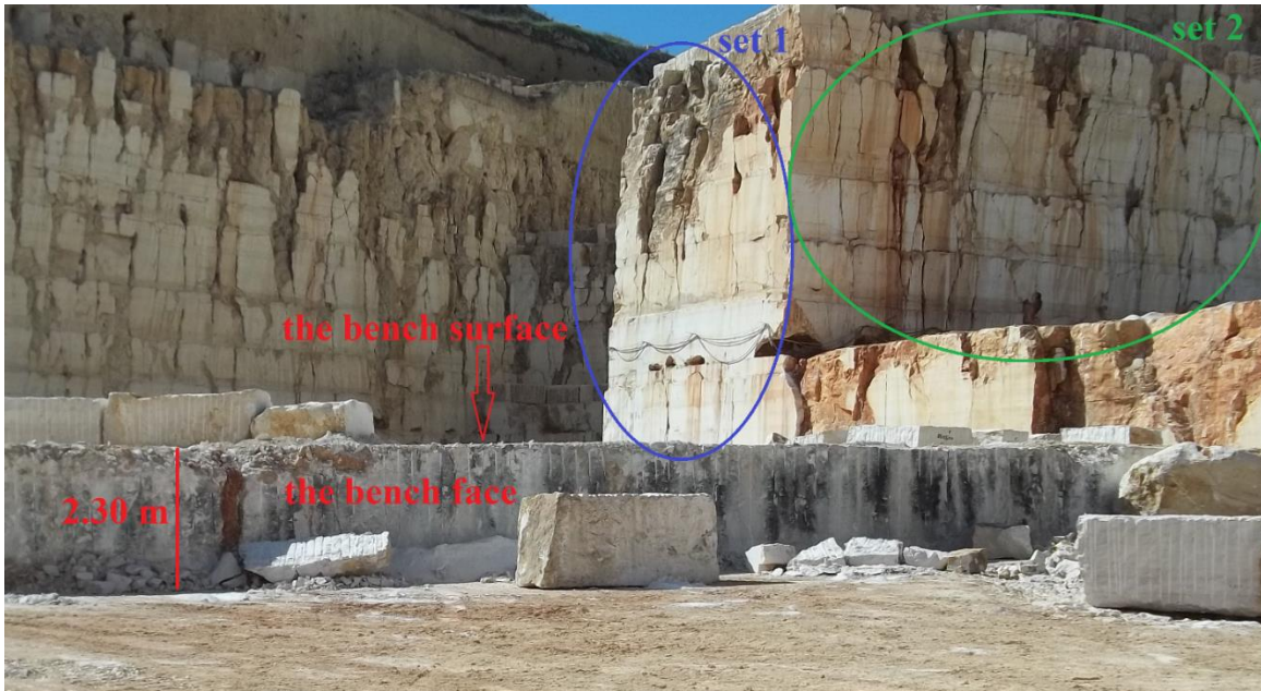
Figure 38: A view of the bench face and highlighting the two sets of fractures.
