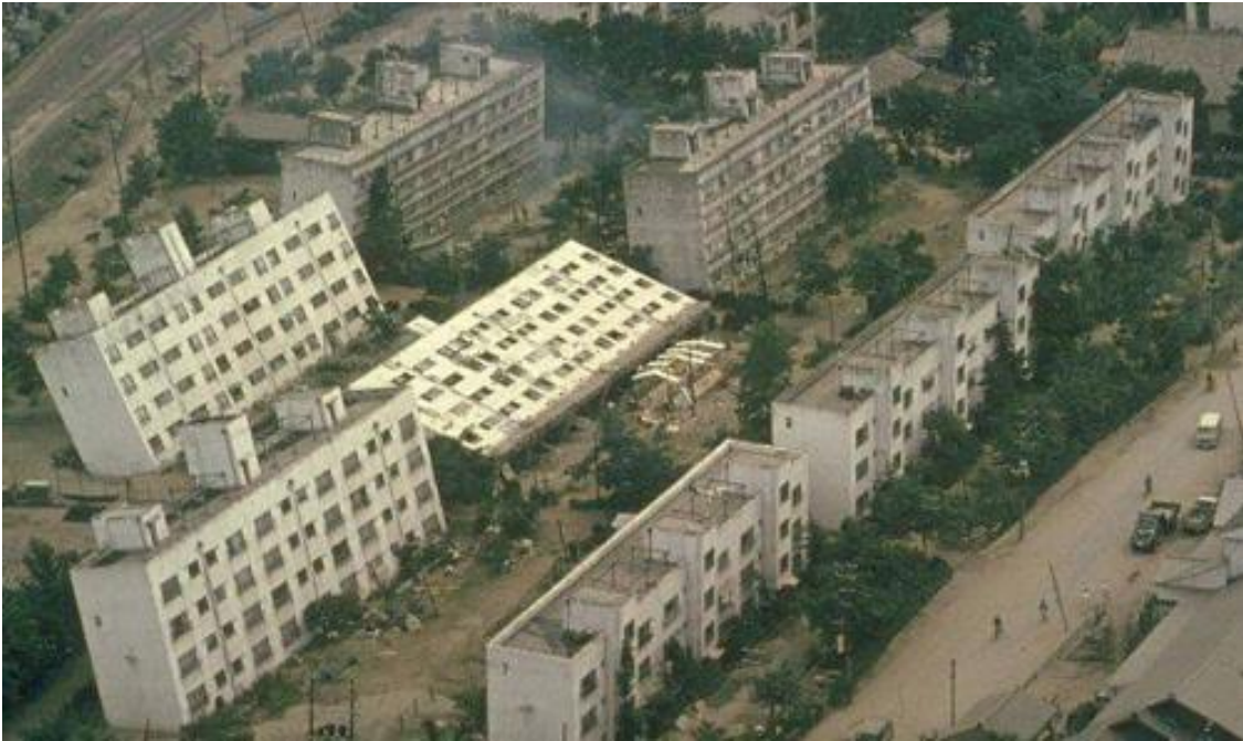
Figure 1.3 Tilting of buildings during the 1964 Niigata earthquake (from Kramer 1996).
