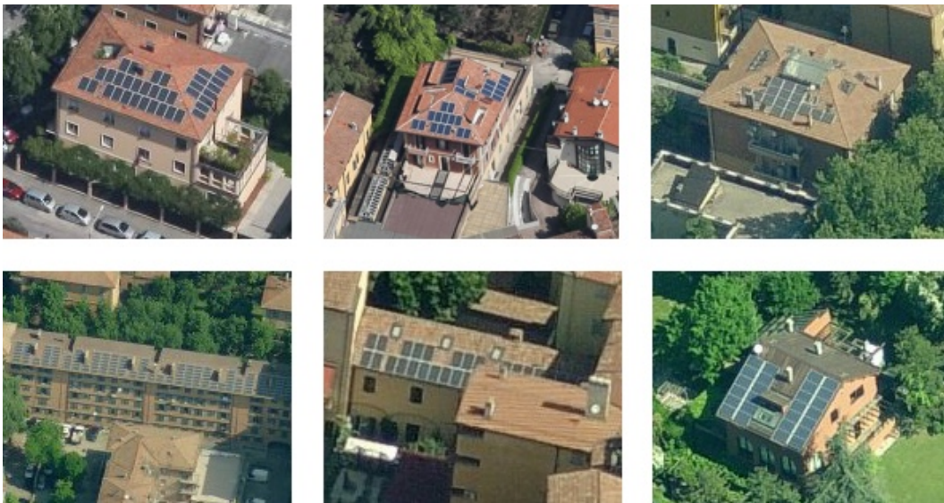
Figure 93: Examples of solar panels placement over complex roofs in the city of Bologna (comune.bologna.it)
