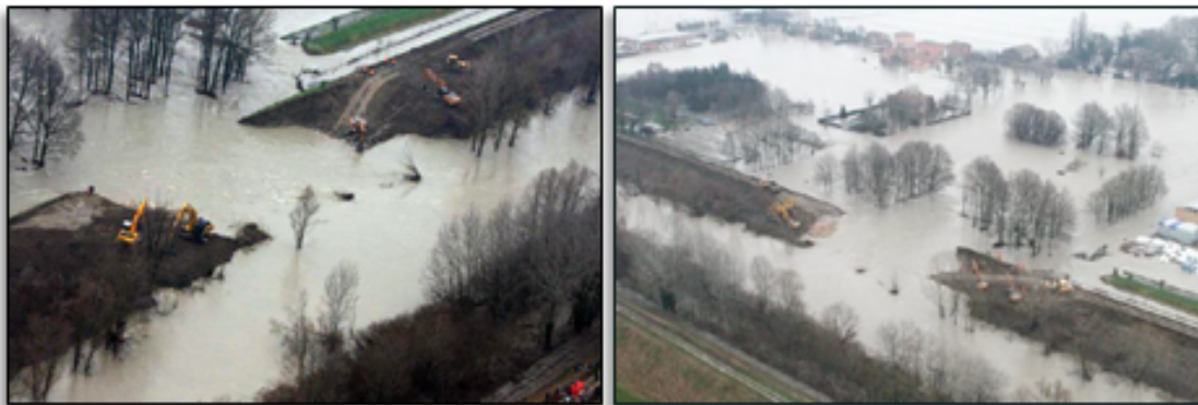
Figure 5.3: Pictures of the breaching point on the right embankment of the Secchia river (sources: www.emiliaromagnameteo.com ; www.nimbus.it ).
