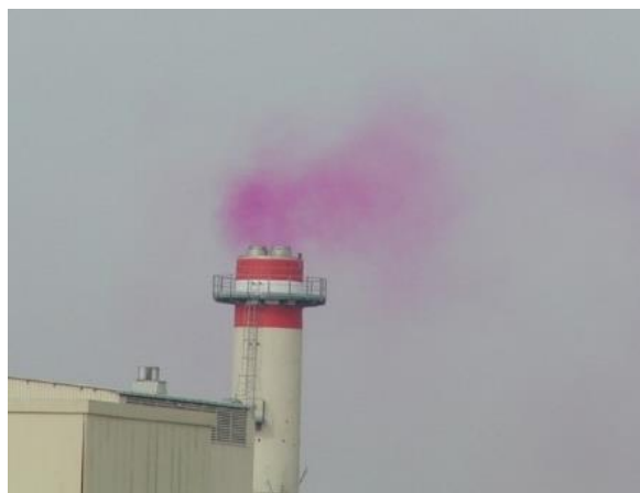
Figure 1.2. Purple-coloured plume emanating from the exhaust stack of the WtE plant in Pisa (Italy) due to hydrogen iodide emission (March 2007).
