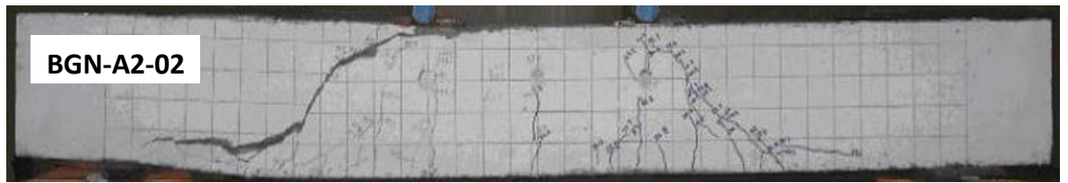
Figure 2.26: Bond/anchorage failure of beam BGN-A2-02
