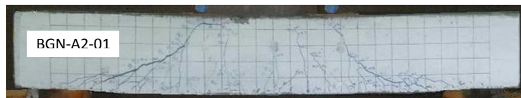
Figure I.3: Crack patterns of beam BGN-A2-01
