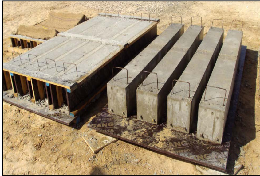
Figure 2.13: Curing process and removing the beams from the formworks
