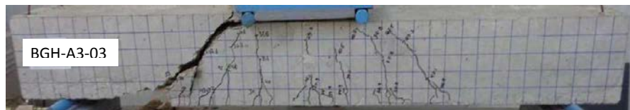
Figure I.9: Crack patterns of beam BGH-A3-03
