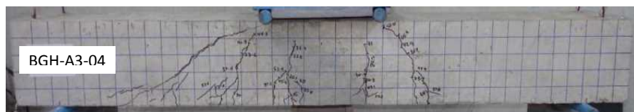
Figure I.10: Crack patterns of beam BGH-A3-04
