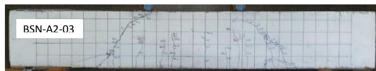
Figure I.5: Crack patterns of beam BSN-A2-03
