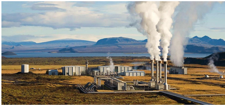
Figure 2.3. Iceland's Nesjavellir geothermal power station. Geothermal plants account for more than 25 percent of the electricity produced in Iceland. Photo: Gretar Ívarsson [8].
