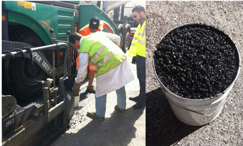
Figure 3.2: Sampling of material during the laying
