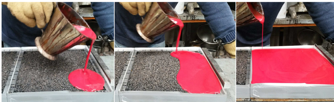
Figure 8.69: Pouring the hot vinamold onto the slab surface
