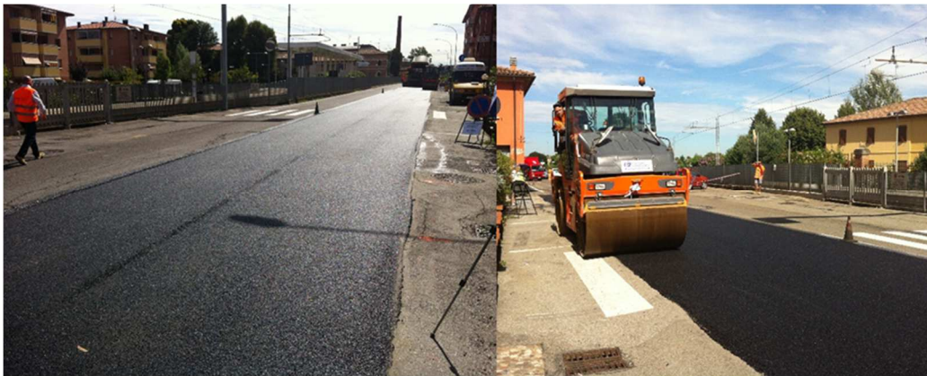
Figure 4.3: Laying and compaction phases of the SMA
