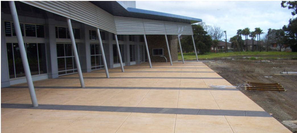
Figure. 2.2 Thomastown Recreation Centre, Thomastown, Australia, E-Crete™ technology used [15].
