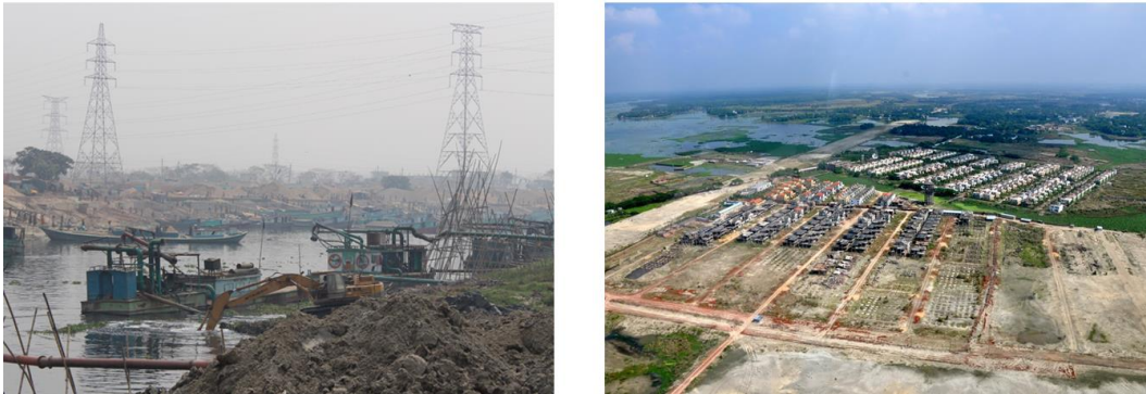
Figure 8 Barges pump sand from the river bed to be distributed across lowlands (left); The Pink City an example of new built-up area in the East of Dhaka (right).
