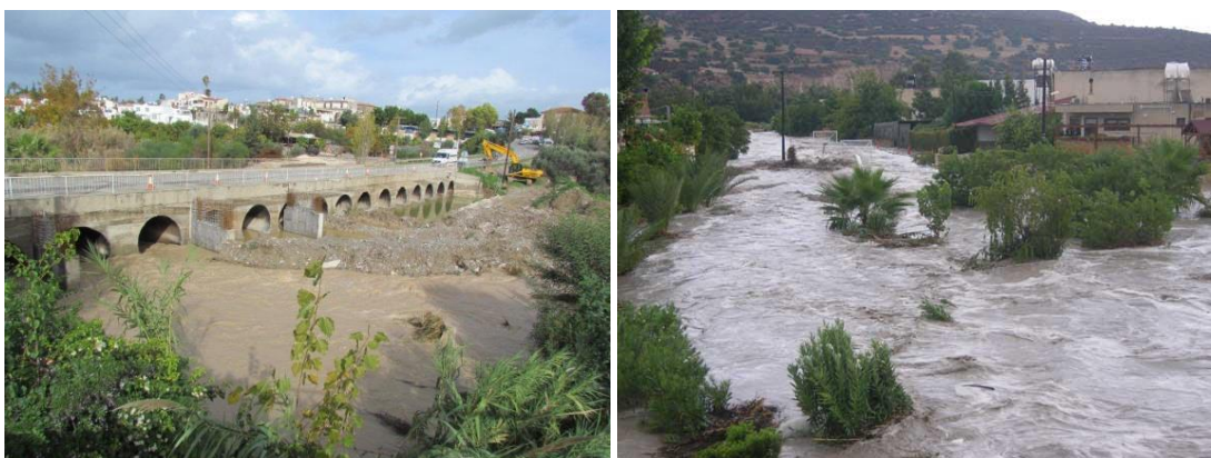
Figure 34 Post-flood debris removing in Polis (Paphos) December 2012 (left); river overflow in Ayios Theodoros (Larnaca) September 2013 (right).
