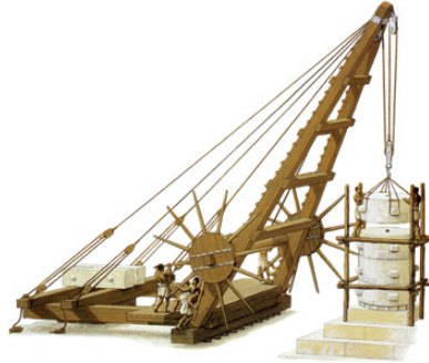
Figure 1.5 – An illustration of a Greek crane during building operations.
