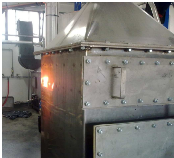
3.6 – Steel carpentry of the new filter.
