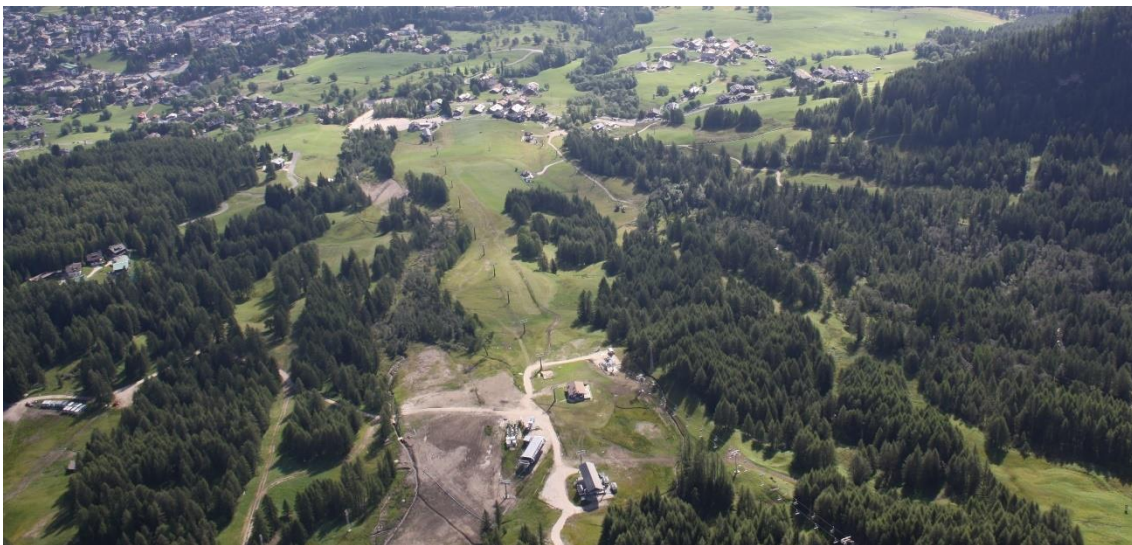
Fig. 54: median track of the landslide with maintenance earth works
