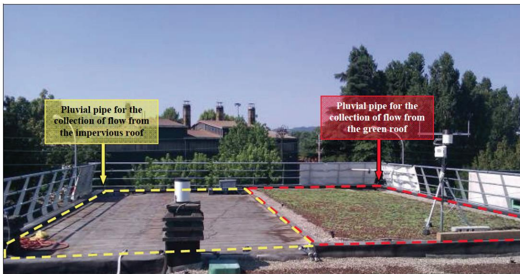
Figure 73: Representation of the green roof and the impervious roof with the bituminous membrane (Maglionico et al., 2014)
