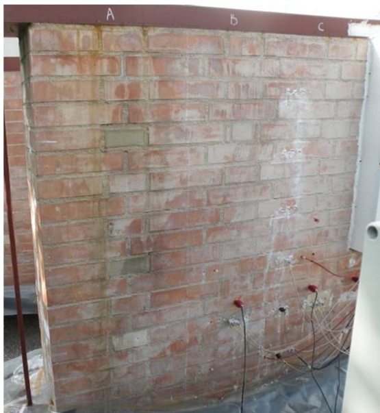
Figure 6.75: Wall PNDB, front side with monitoring sensors, 3rd May 2011
