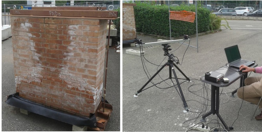
Figure 6.100: Wall PNDD, rear side, October 2013 and testing set-up
