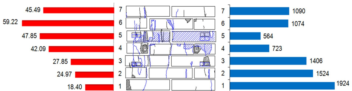
Figure 7.16: Small wall I, after mechanical compression test: values of sonic signal attenuation (left) and direct velocity (right) on each masonry course
