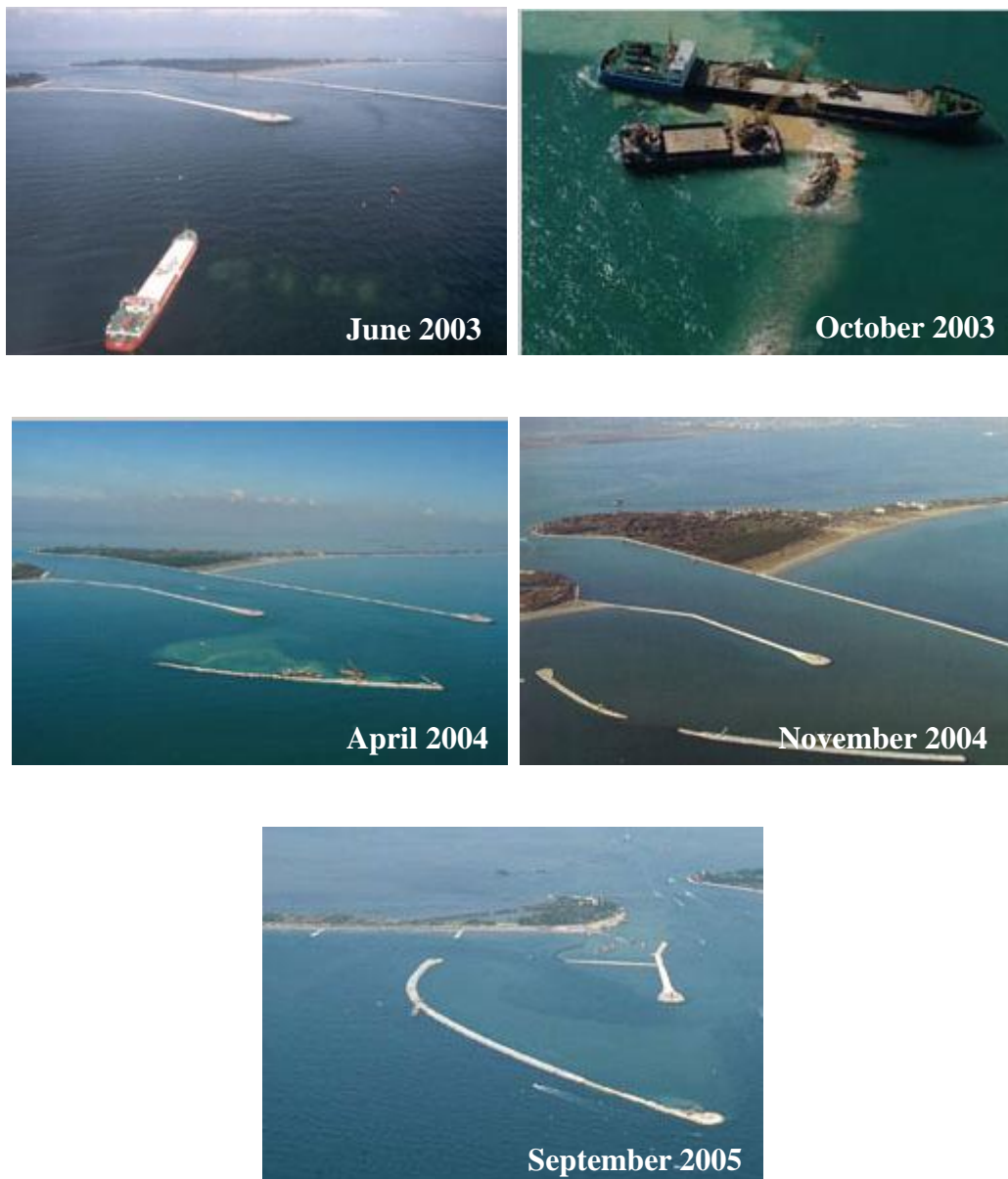
Figure 7.18: Construction history of the breakwater in the Malamocco Inlet (images taken from the website salve.it )
