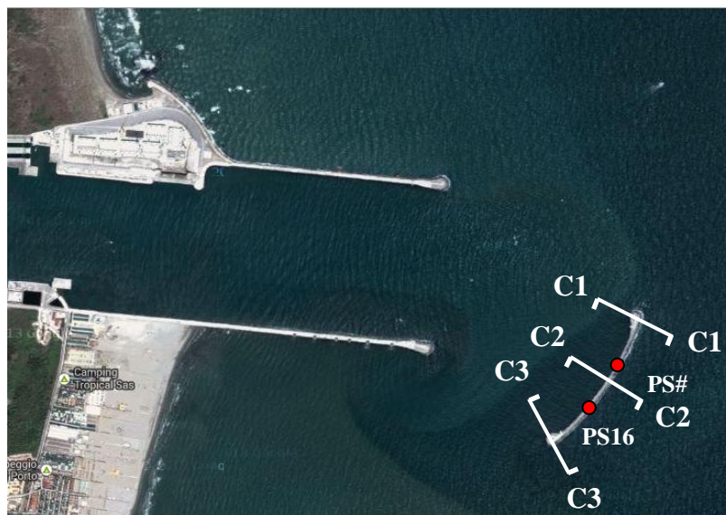
Figure 7.25: Location of the examined cross-sections in the Chioggia breakwater and location of radar reflectors (satellite view)
