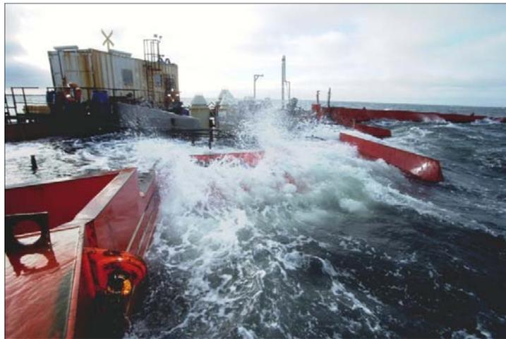
Figure 11: Wave overtopping of the Wave Dragon prototype,[60].
