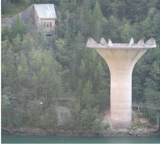
Figure 136: Example of spillway designed according Lazzari's profile, [131]
