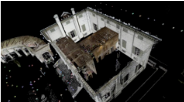
Figure 3.1. Camera positions and dense points of Villa Badoer obtained by SfM techniques. The entrance hall and the exterior walls of the villa are reconstructed in the same model without further registration.
