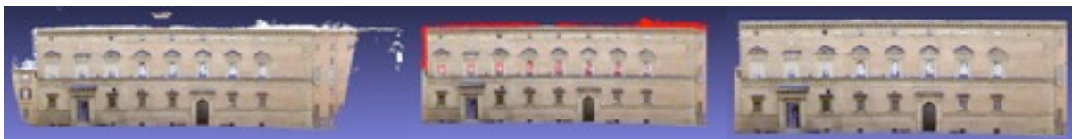
Figure 2.13. Points cloud cleaning. Left: Original points cloud; Middle: cleaning by vertex RGB color filter. Noisy white points on the upper edge of the facade ' R > 245 ' are selected and removed. Right: points cloud after cleaning
