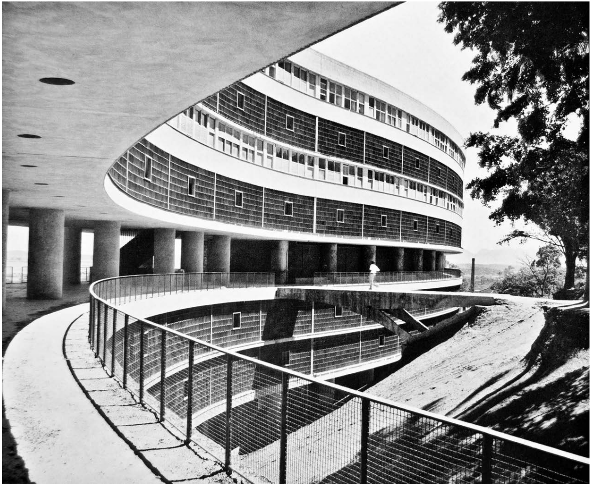
Fig. 9. The Pedregulho social complex, by Affonso Eduardo Reidy
