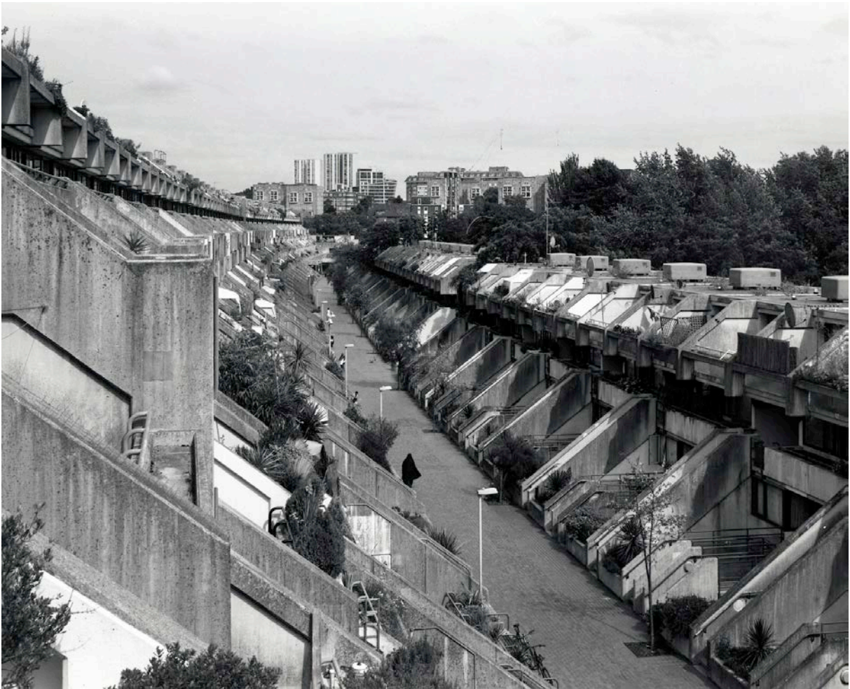
Fig. 8. Alexandra Road Estate, 1968.
