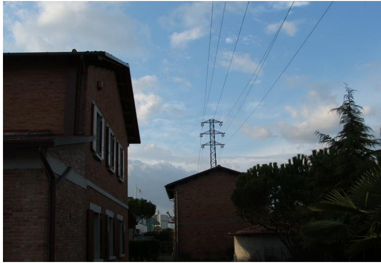
Figure 6.9: Photo of the double-circuit power line close to the measurement point.
