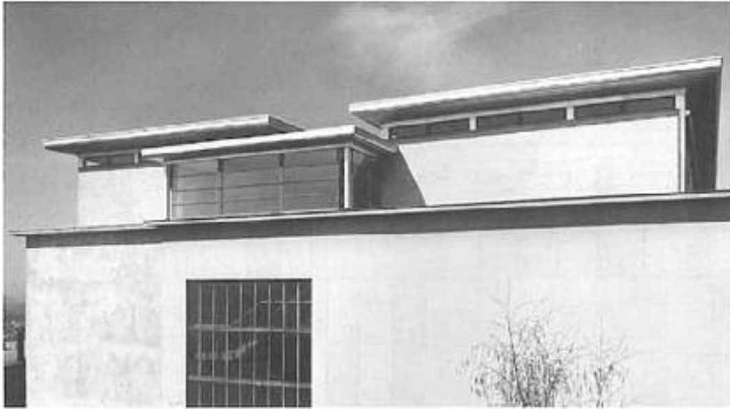
South elevation of the new story
