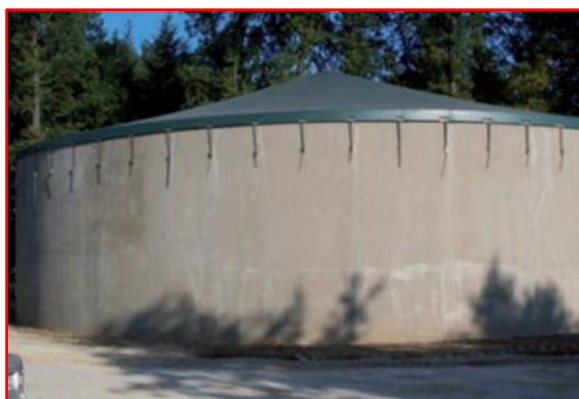
Fig. 2.46: Covered digestate storage tank (as cited in Lukehurst et al. , 2010)
