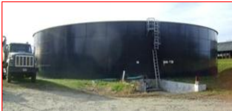
Fig. 2.15: Manure slurry tank (as cited in Department of Environmental Protection, 2009 )
