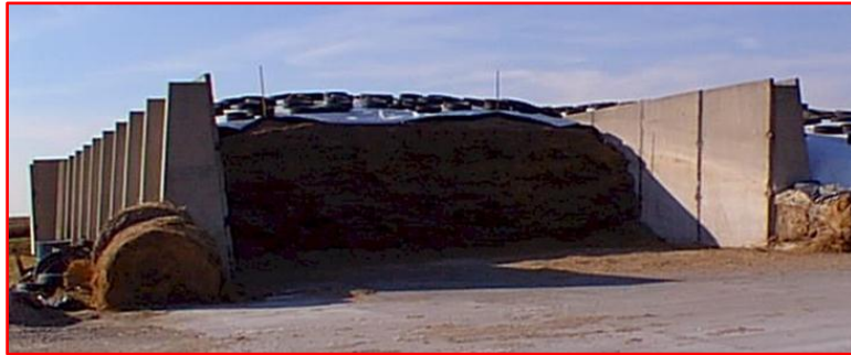
Fig. 2.14: Bunker silo, made of concrete and silage is covered by plastic foils (as cited in Purdue Dairy Page, 2012 )
