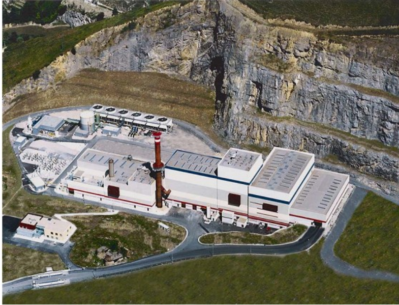
Figure 1 : A picture of Zabalgardi integrated WTE-CC power plant [16].
