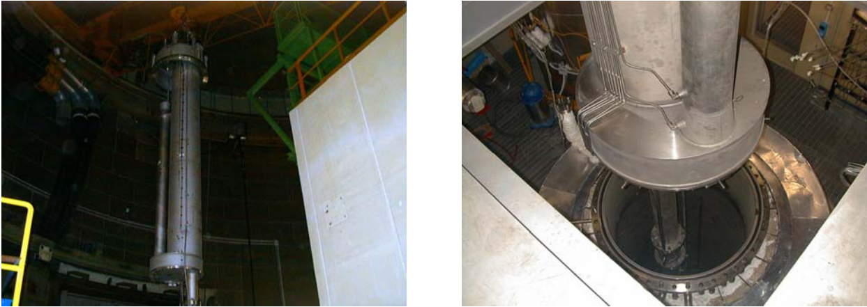
Figure 2-1- Handling of the test section N° 2 in the PEC building and inserting it inside the main vessel.
