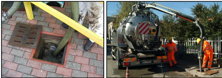
Figure 2.5 - Gully pot cleaning operations
