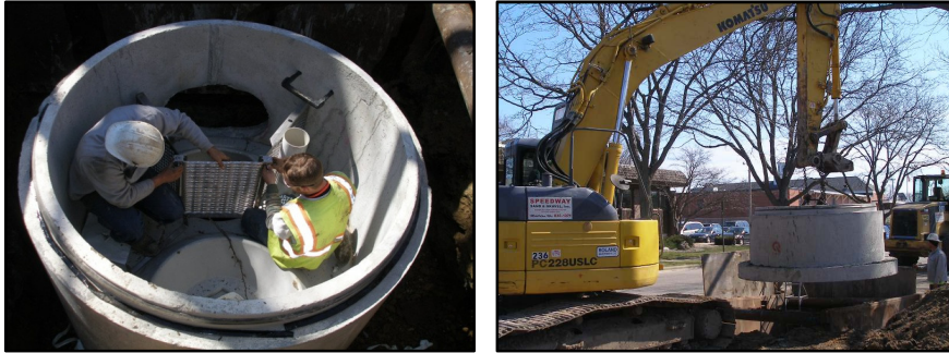
Figure 3.1 - Installation of an hydrodynamic separator
