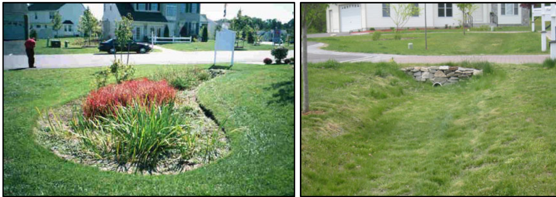
Figure 1.5 - Residential on-lot rain garden (left); grassed swale(right)
