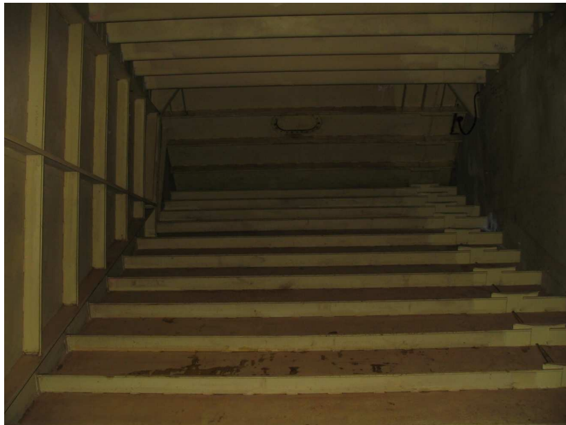
Figure 5.2.3 View of the inside of the deck.
