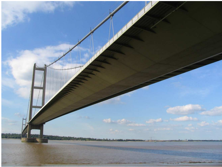
Figure 5.2.4 The box-girder shape of the deck of Humber Bridge
