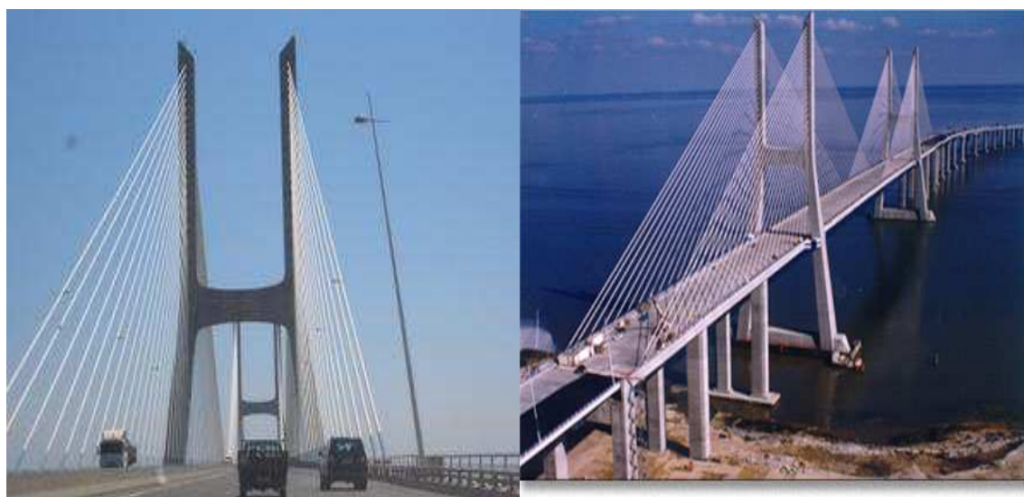
Figure 3.3.1 Cable-stayed component of Vasco da Gama Bridge
