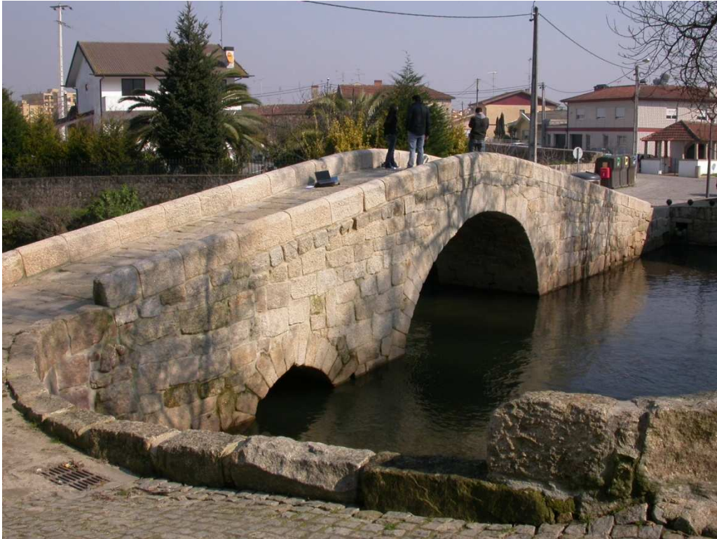
Figure 4.5.1 General view of the bridge
