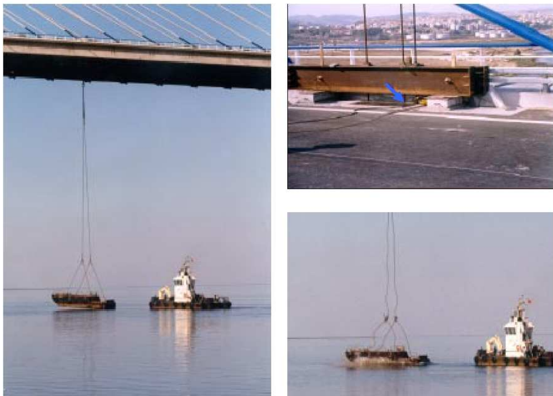
Figure 3.3.2 Eccentrically suspended barge, its cutting and release
