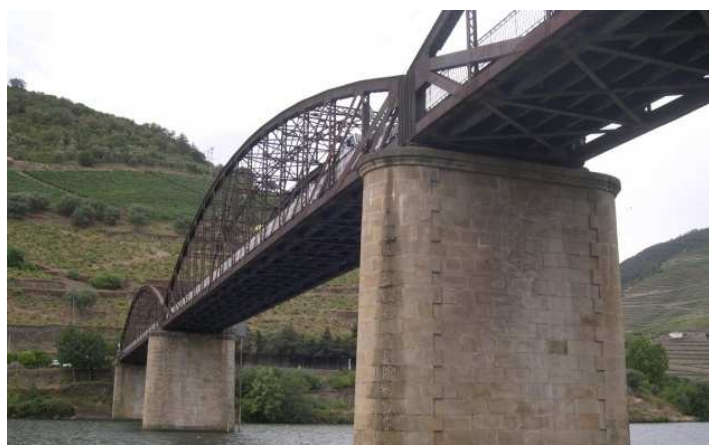
Figure 3.4.1 View of Pinhão Bridge
