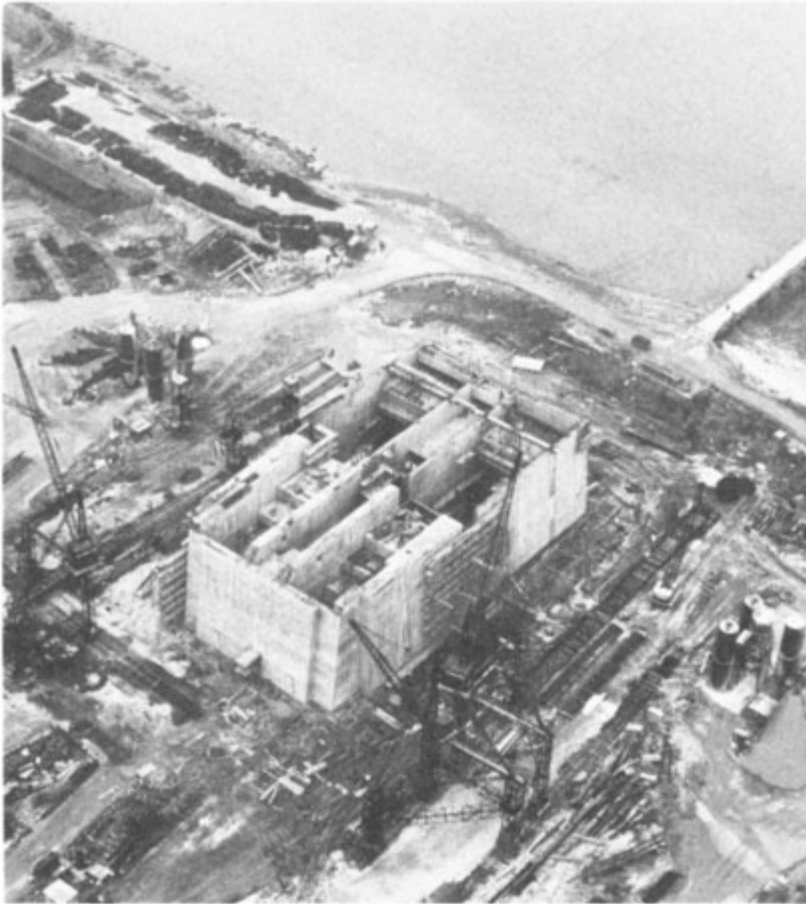
Figure 5.2.6 Barton anchorage nearing completion.
