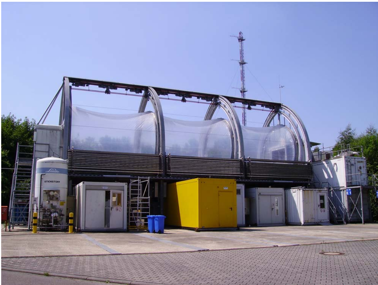
The outdoor chamber SAPHIR in Jülich, Germany.
