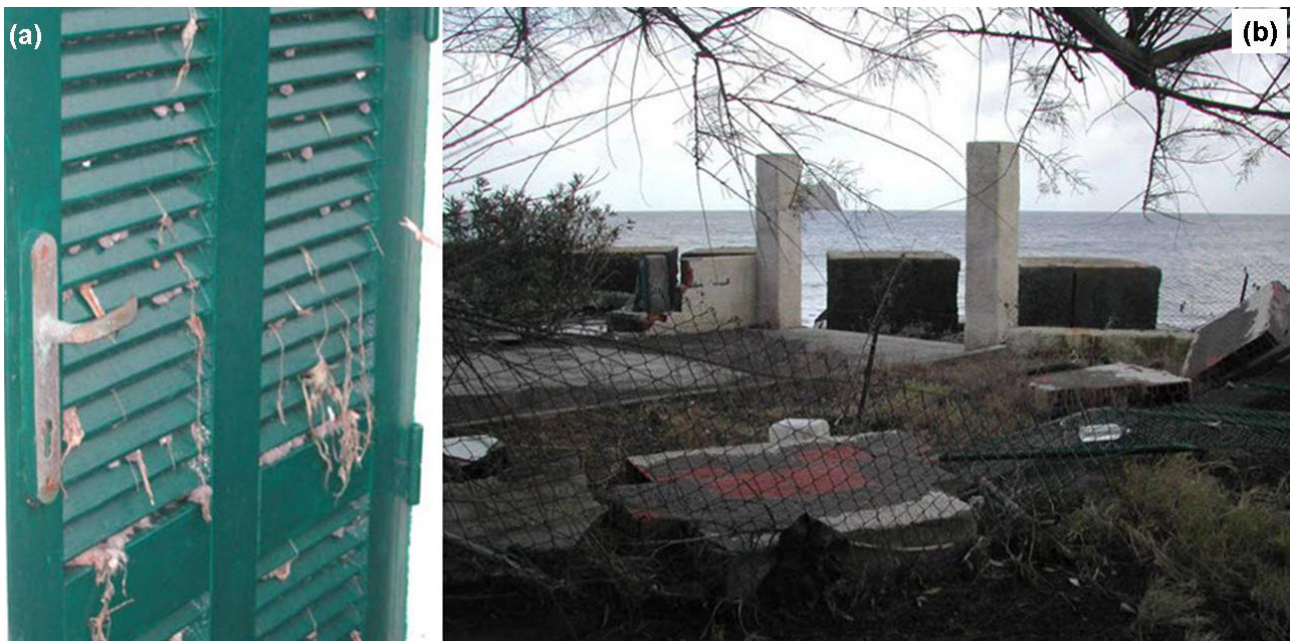
Figure 11. Two images of building #4 (Punta Lena, Stromboli-Figure 6), taken after the 2002 tsunami. Figure 11(a) shows a door on the seaward wall of the building. The inundation did not break it down, but penetrated indoor through the shutter openings and flooded the ground-floor. The building was protected by the vegetation in the front garden (Figure 11b), some concrete works (a small wall and a table) and by the costal defences along the shoreline (concrete cubic rocks). The PTVA-3 Model classified this building as having a “low” RVI.
