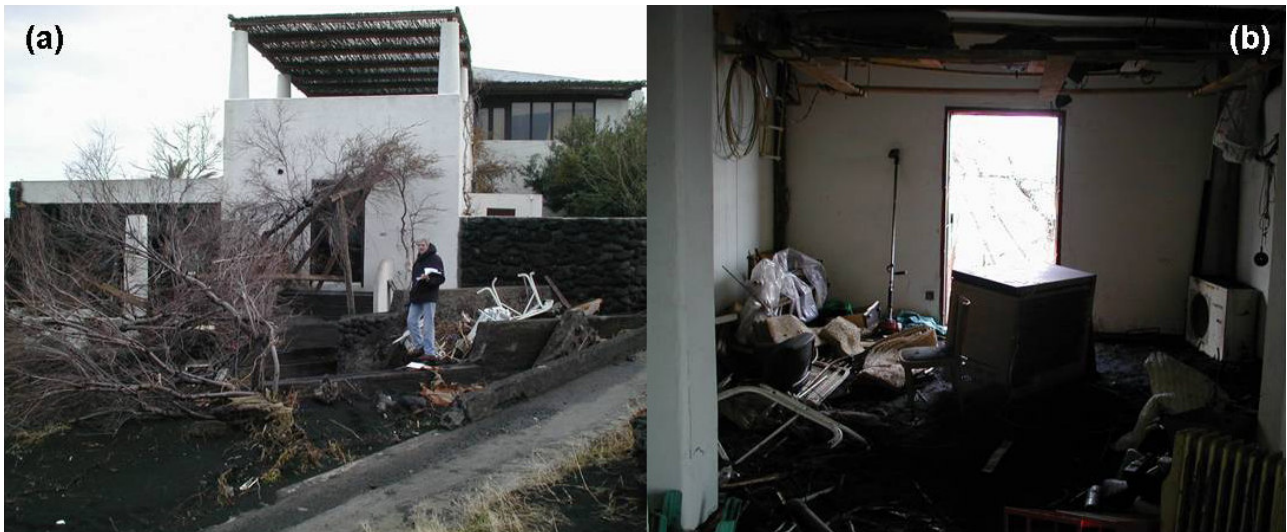
Figure 9. Pictures of building #2, at the eastern end of Ficogrande (Stromboli – Figure 5), taken after the 2002 tsunami. Figure 9(a) shows a view of the building from north-west. Figure 9(b) shows damage to the interiors. The PTVA-3 Model classified building #2 as having an “average” RVI score.
