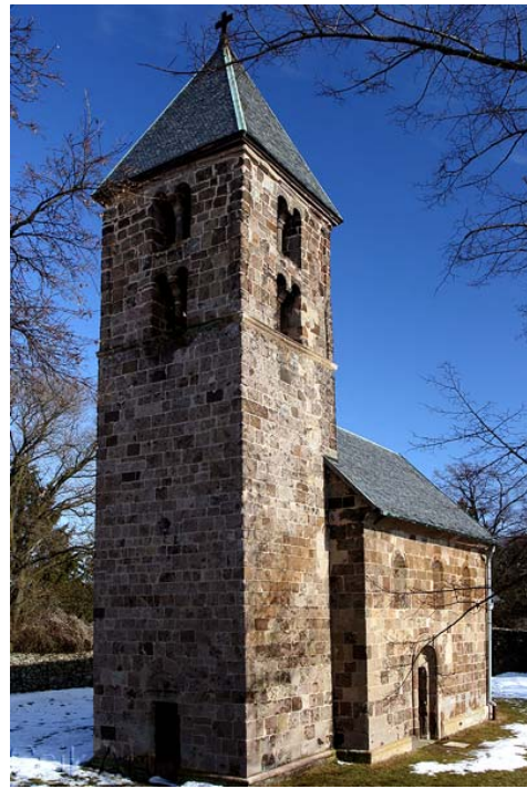
Fig. 3.11 The church of Nagybörzsöny constructed of trachite in the 13 th century. Photo from http://wiki.utikonyvem.hu/
