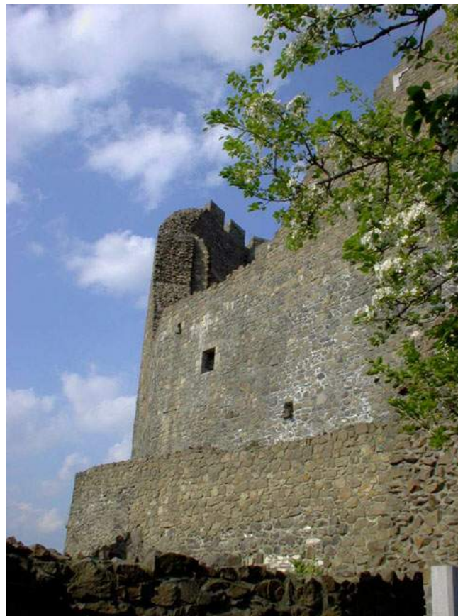
Fig. 3.12 The castle of Hollókő is one member of the defence chain built in the 13 th -17 th centuries using local stone material, mainly andesite
