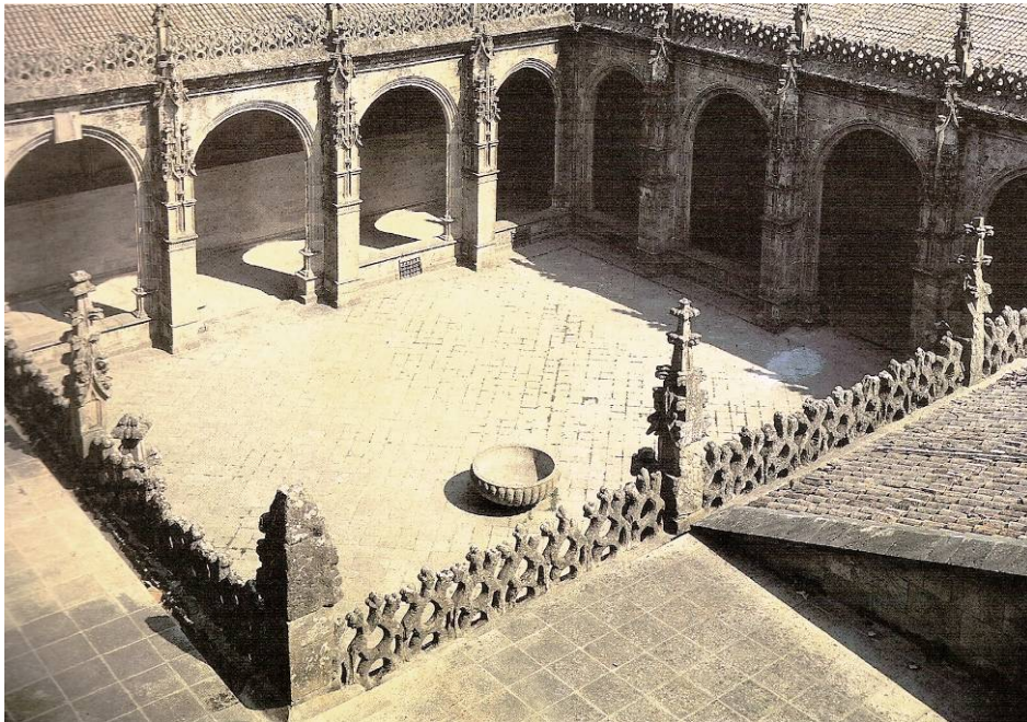
Fig. 3.8. The cloister of the Cathedral of Santiago is also constructed of granite. Photo from Sarthou and Navascués, 1990
