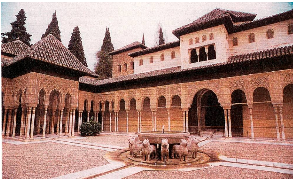
Fig. 3.2. One of the most famous examples of the monumental use of the Macael marble: the columns and the lions of the Patio de los Leones of the Alhambra (Granada, Spain). Photo from Sáez Pérez 2003
