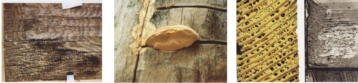
(a) Carbonized and rotted wood (b) Fungal attack (c) Xylophagous insect attack
