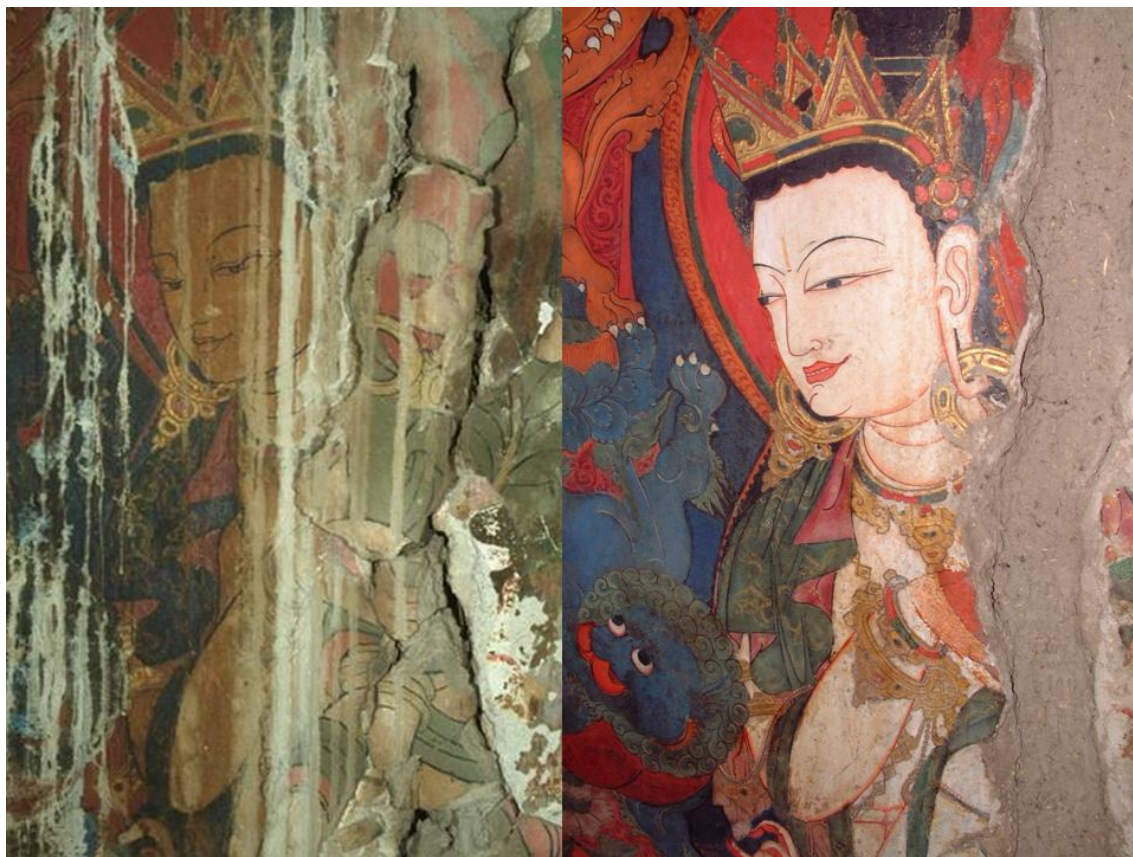
Figure 7.12: Mural painting from Thubchen Lakhang temple, before and after restoration (and after removal of over-paintings), showing the evidence that water has run down the mural painting for years leaving a visible layer of clay on the surface of the painting.
