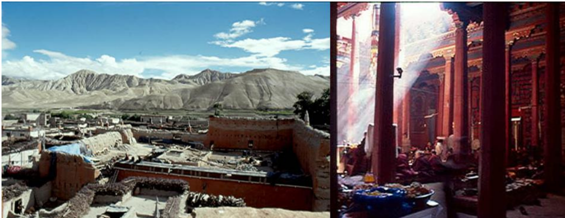
Figure 7.6: Pictures of the Thubchen Lakhang monastery seen from the outside and the decorated and painted hall after reconstruction.
