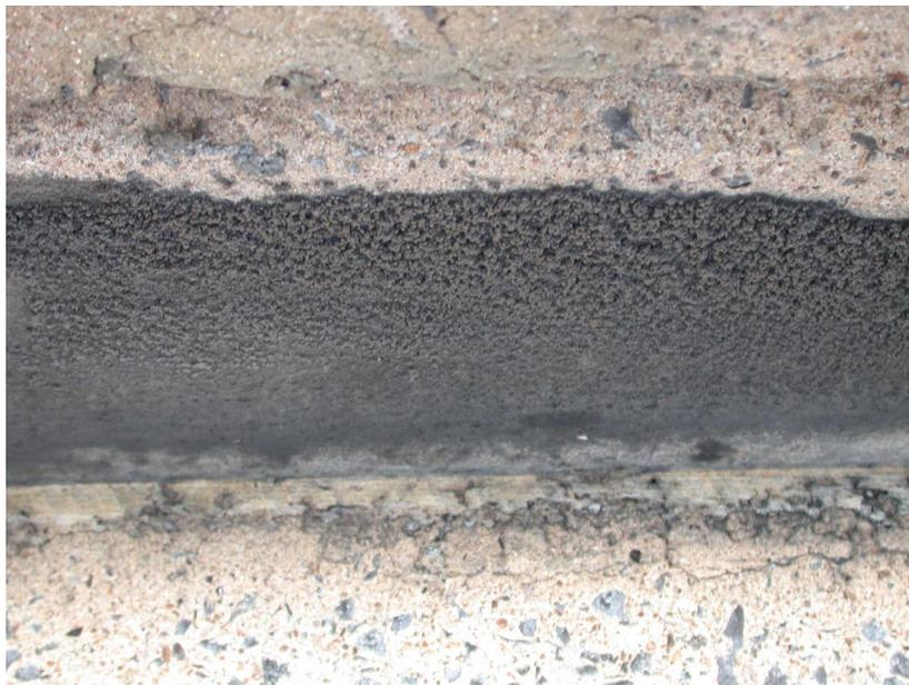
**Figure 3.4.** Centennial Hall, black thick crust in area protected from rain run-off.
