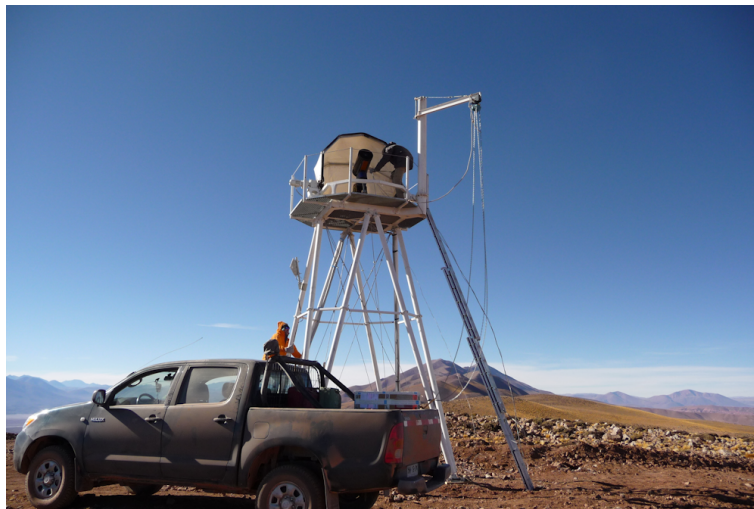
Figure A.5: Astronomical Site Monitor installation at Macon in May 2008.
