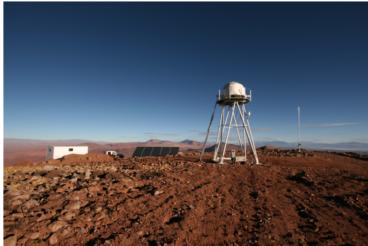
Figure A.7: This picture shows the typical Astronomical Site Monitor installations. From left to right: a hut for nighttime work, solar panels for energy providing, the 5 m MASS-DIMM tower and the automatic weather station. The picture has been taken at Macon in July 2008.
