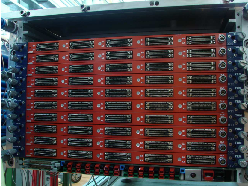
Figure 2.13: Front view of the ALICE TOF crate with 10 TRM boards installed.
