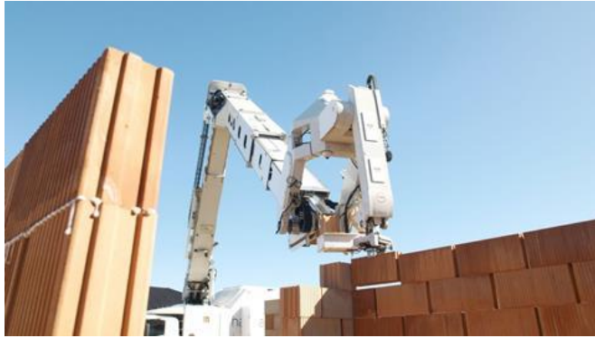
(c) Automated laying of commercial blocks (Source: Fastbrick Robotics).
