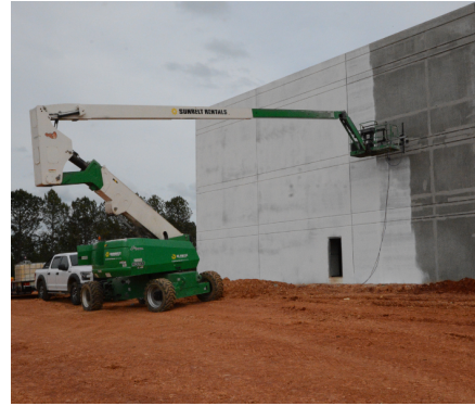
(d) Robotic construction painting (Source: PaintJet).
