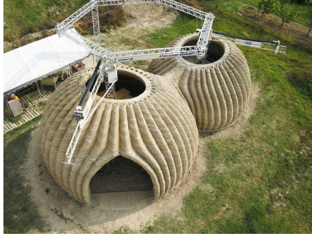
(a) TECLA Crane WASP, 3D printed housing (Source: WASP).
