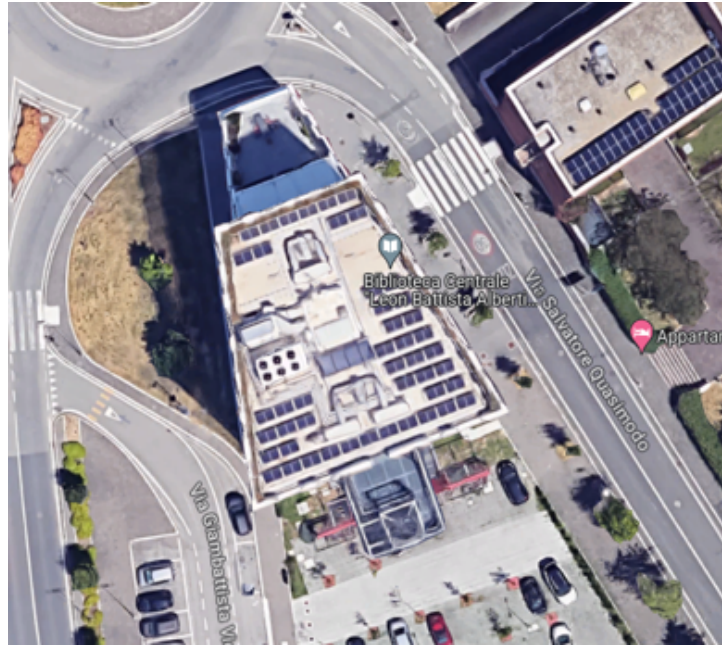
Figure 3.43: Picture of the university building roof with the installed PV arrays.
